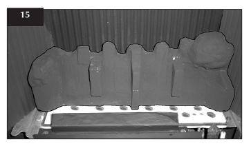
8.8 Place the front coal centrally in the channel at the front of the tray. The relationship between the front coal and the flame baffle is shown, Diagram 16
