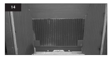
8.7 Position the flame baffle centrally on the tray and ensure the stepped lower edge engages against the rear edge of the burner skin, Diagram 15
